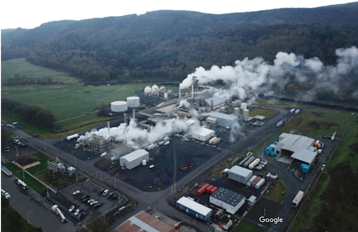
DYNO NOBEL INC. CHEMICAL PLANT (YES THAT NOBEL) DEER ISLAND, OREGON, USA ALONG THE COLUMBIA RIVER. PRODUCES AGRICULTURAL CHEMICALS INCLUDING AMMONIUM NITRATE.
